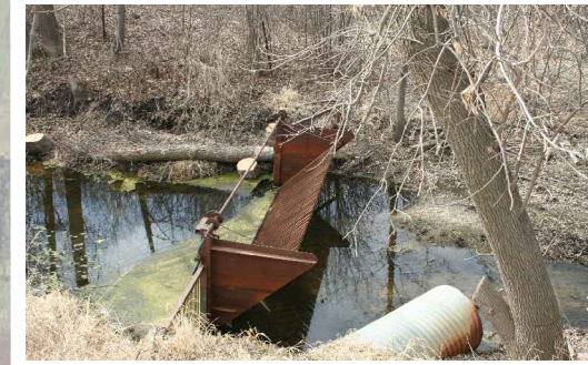
PHOTO C. FISH BARRIER INSTALLATION EXAMPLE 1
