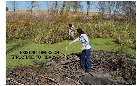
PHOTO B. EXISTING DIVERSION TO BE REMOVED
