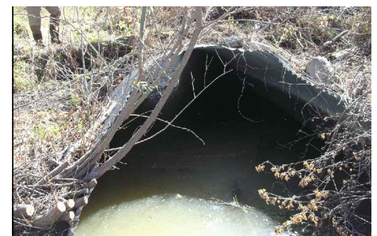
PHOTO A. EXISTING CULVERT TO BE REMOVED
