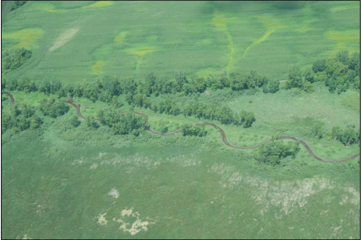
Figure 1: Aerial of restored low flow river channel
