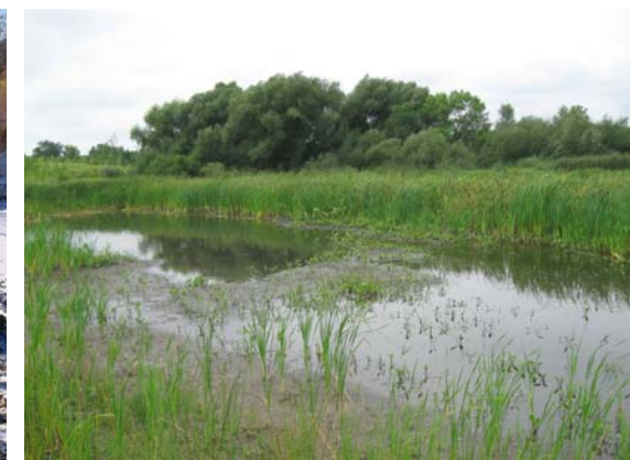
Before and after: Segner Pond in December 2007 and August 2009. This treatment wetland was constructed on the inlet to Cedar Lake to remove phosphorus from water before it enters the lake.
