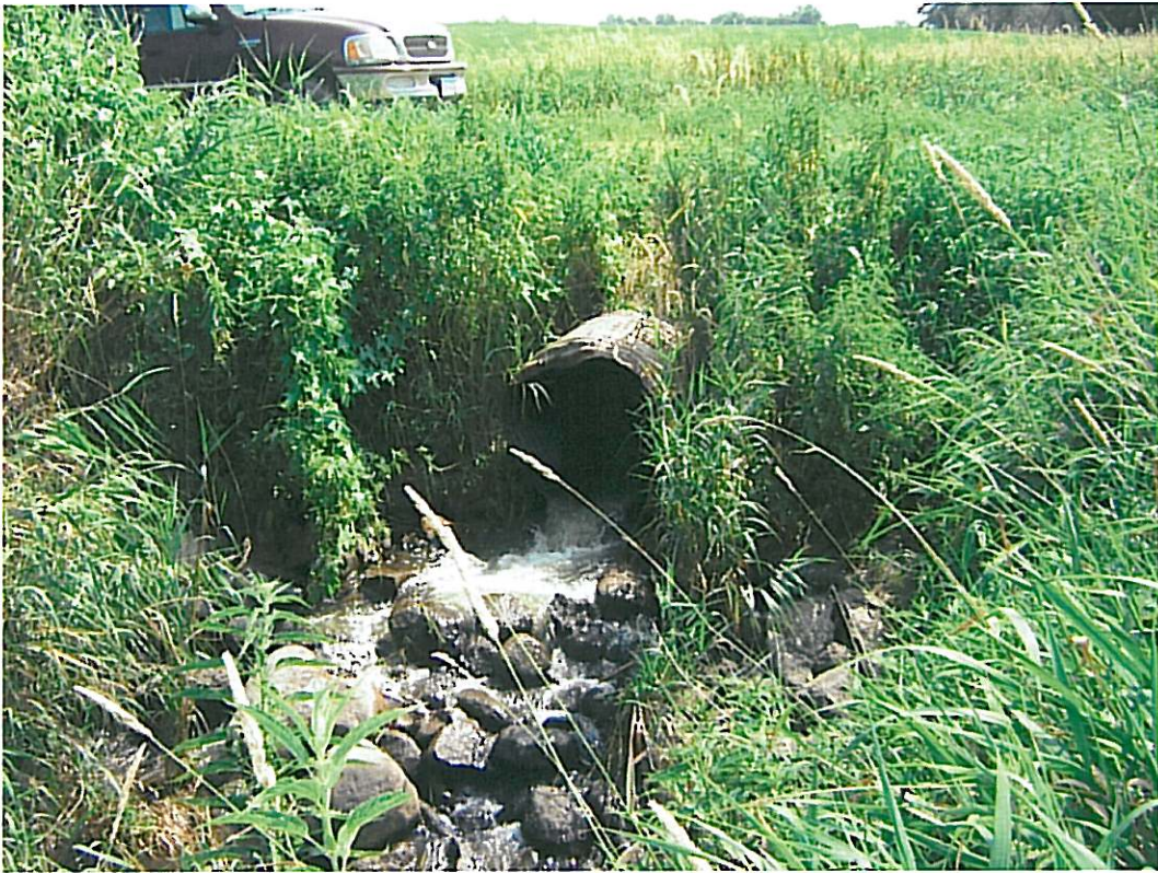
Henshaw Lake Outlet Channel crossing at field road
