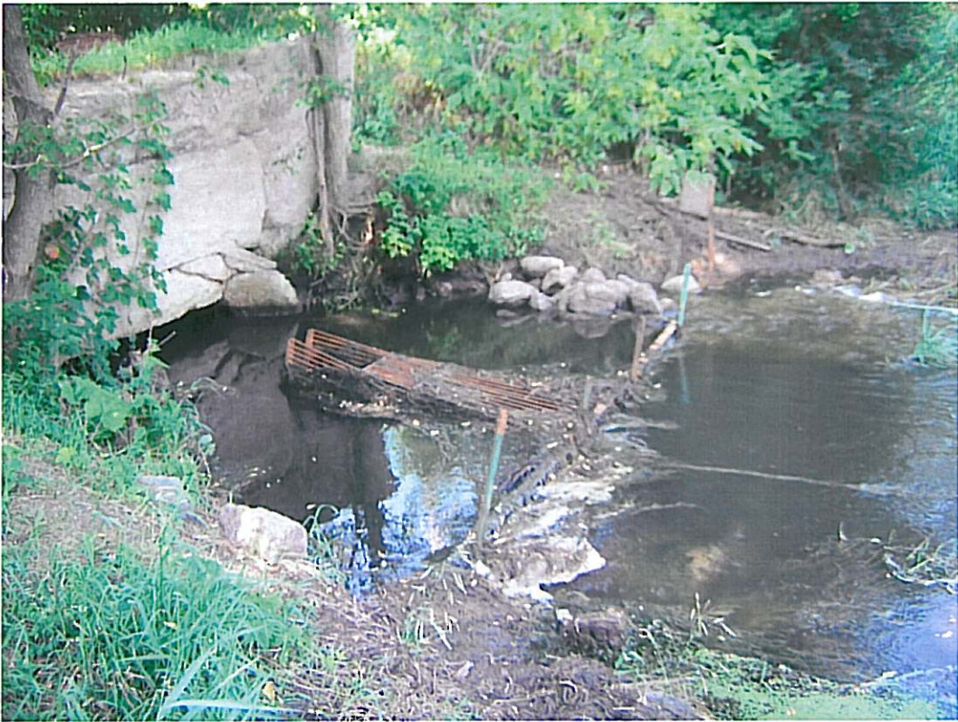
Existing Fish trap structure on downstream side of Old Hwy 55
