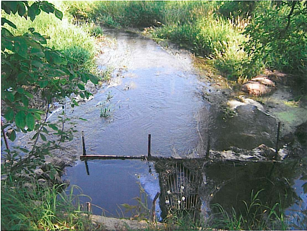
Looking downstream at existing fish trap structure
