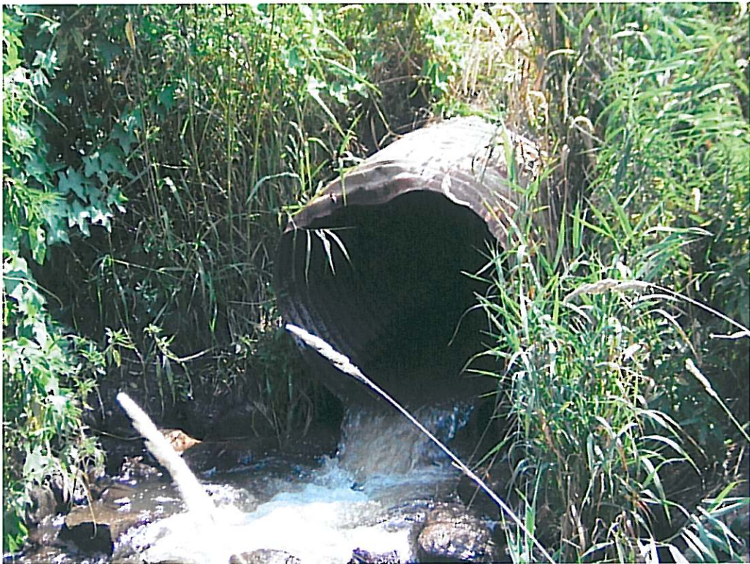
Culvert under field road at Henshaw Lake outlet.
