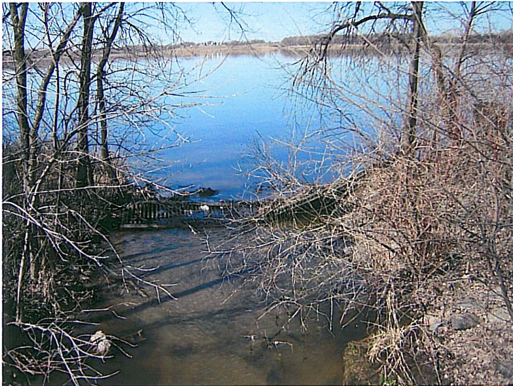
Fish barrier structure at Swartout outlet.
