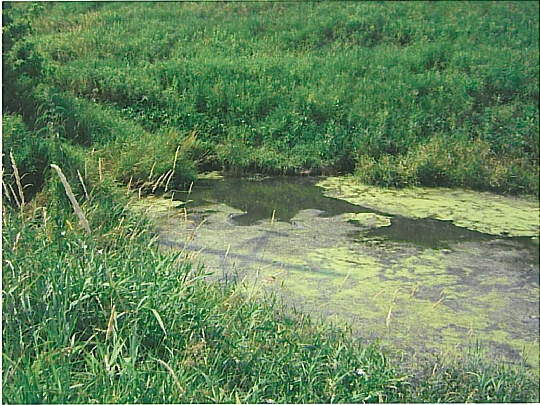
Downstream end of culvert under Hwy 55
