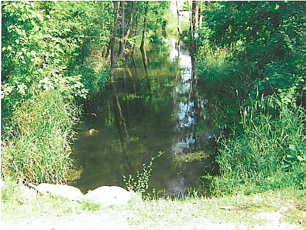
Channel on downstream side of Illsley Ave crossing
