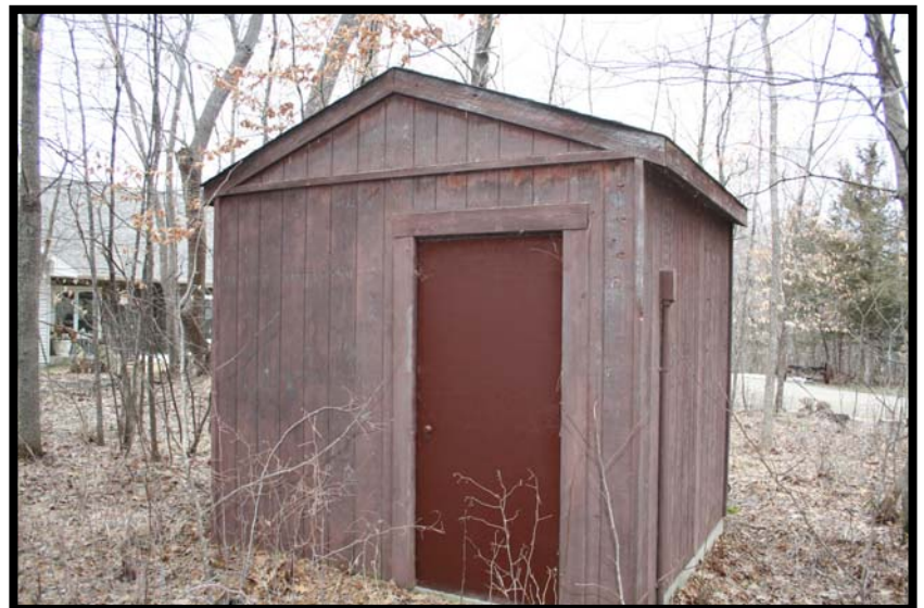
Photo 8-Lake Marie Aerator Building
