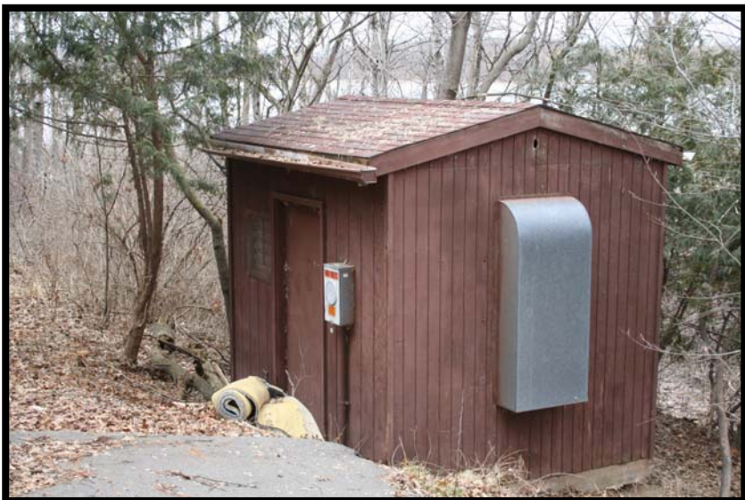
Photo 7-Lake Augusta Aerator Building
