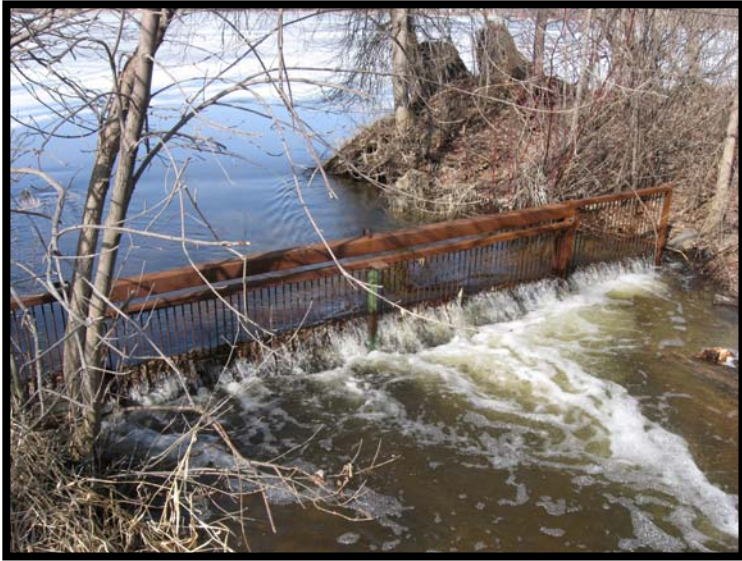
Photo 17-Swartout Outlet Fish Barrier
