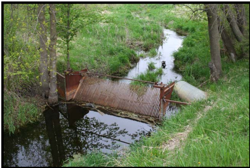
Photo 19-Illsley Ave Fish Barrier
