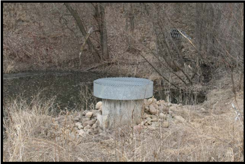
Photo 13-Lake Augusta Sedimentation Pond Riser Structure
