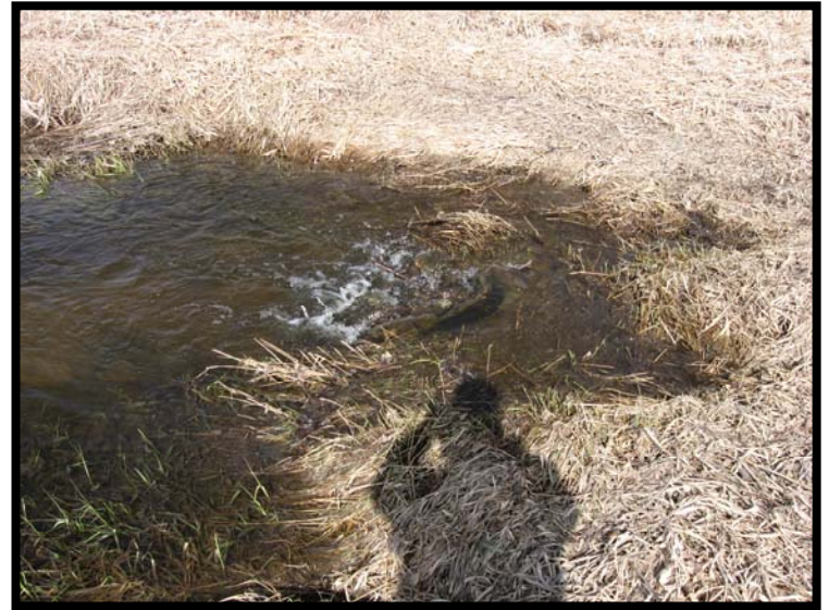
Photo 2-Watkins Wetland Diversion Structure
