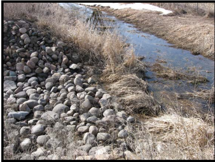
Photo 1-Watkins Wetland Overflow Berm
