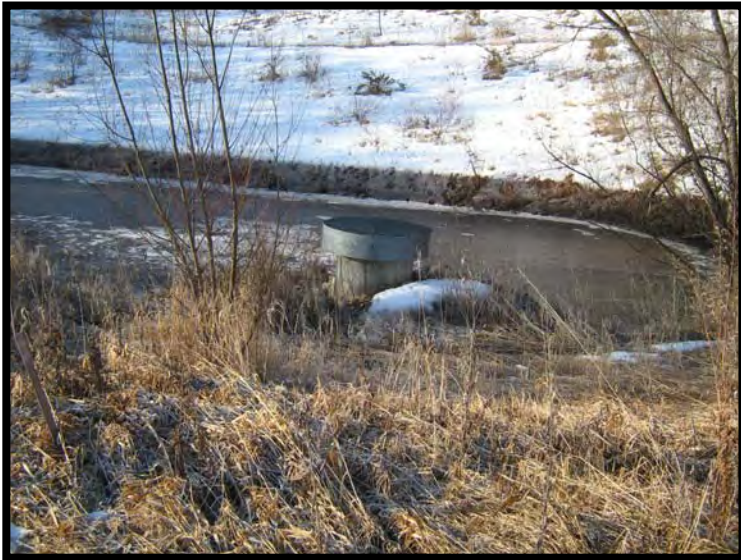
Photo 11-Lake Augusta Erosion Control Project Riser Structure
