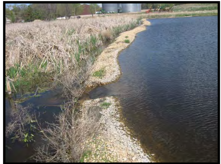
Photo 20-Segner Pond Limestone Berm
