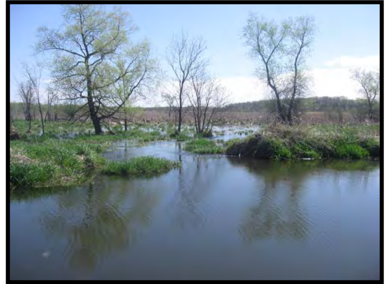
Photo 6-Kingston Wetland Berm Washout
