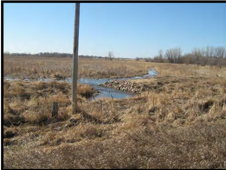
Photo 1-Watkins Wetland-North Overflow Berm installed in 2008.
