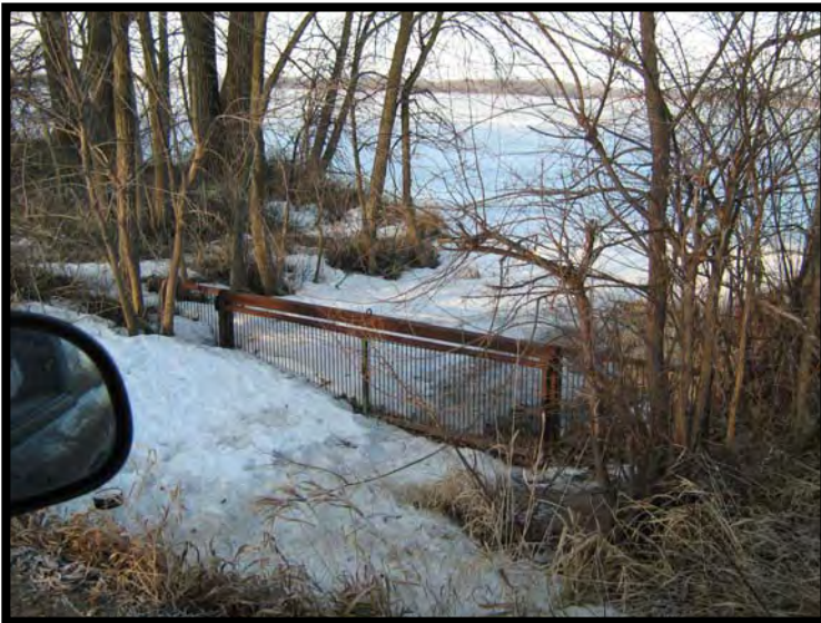
Photo 15-Swartout Outlet Fish Barrier
