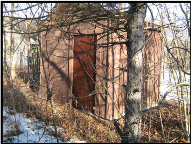
Photo 7-Lake Marie Aerator Building
