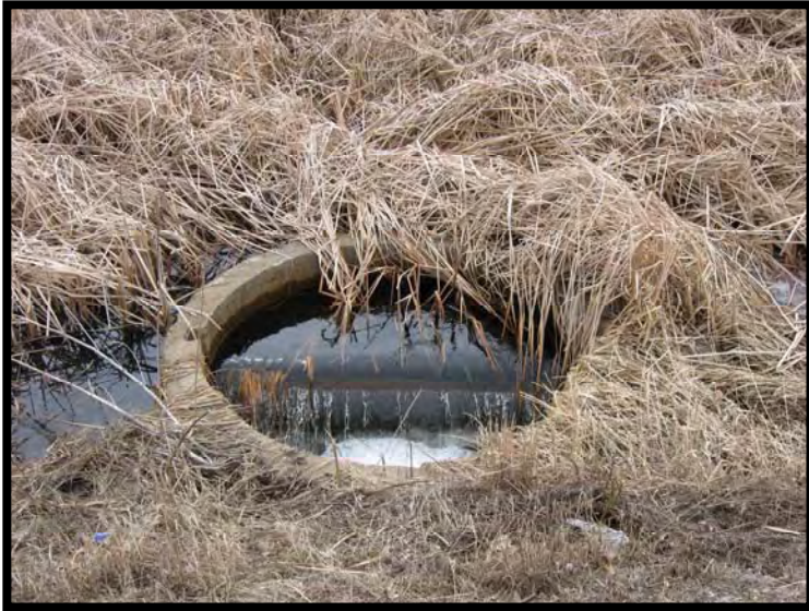
Photo 9-Annandale Wetland Outlet Structure
