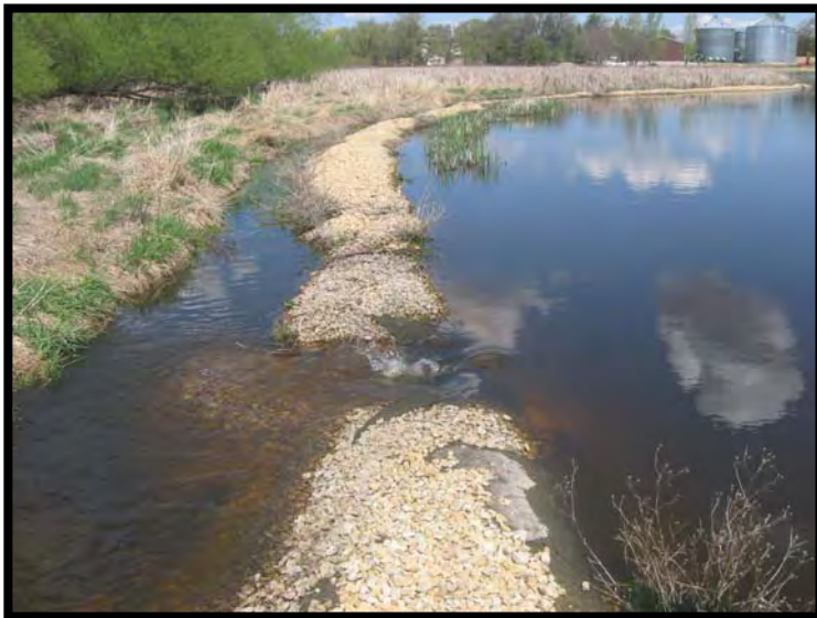
Photo 19-Segner Pond Limestone Berm
