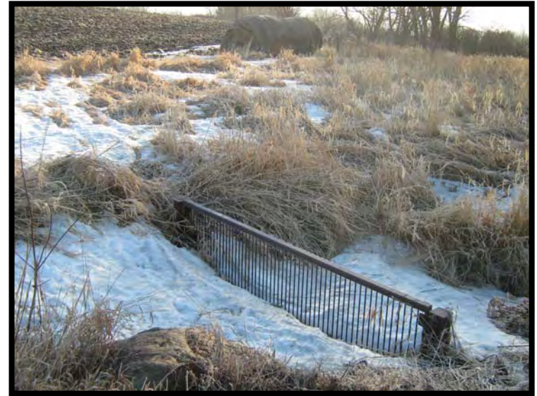
Photo 14-Henshaw Lake Fish Barrier
