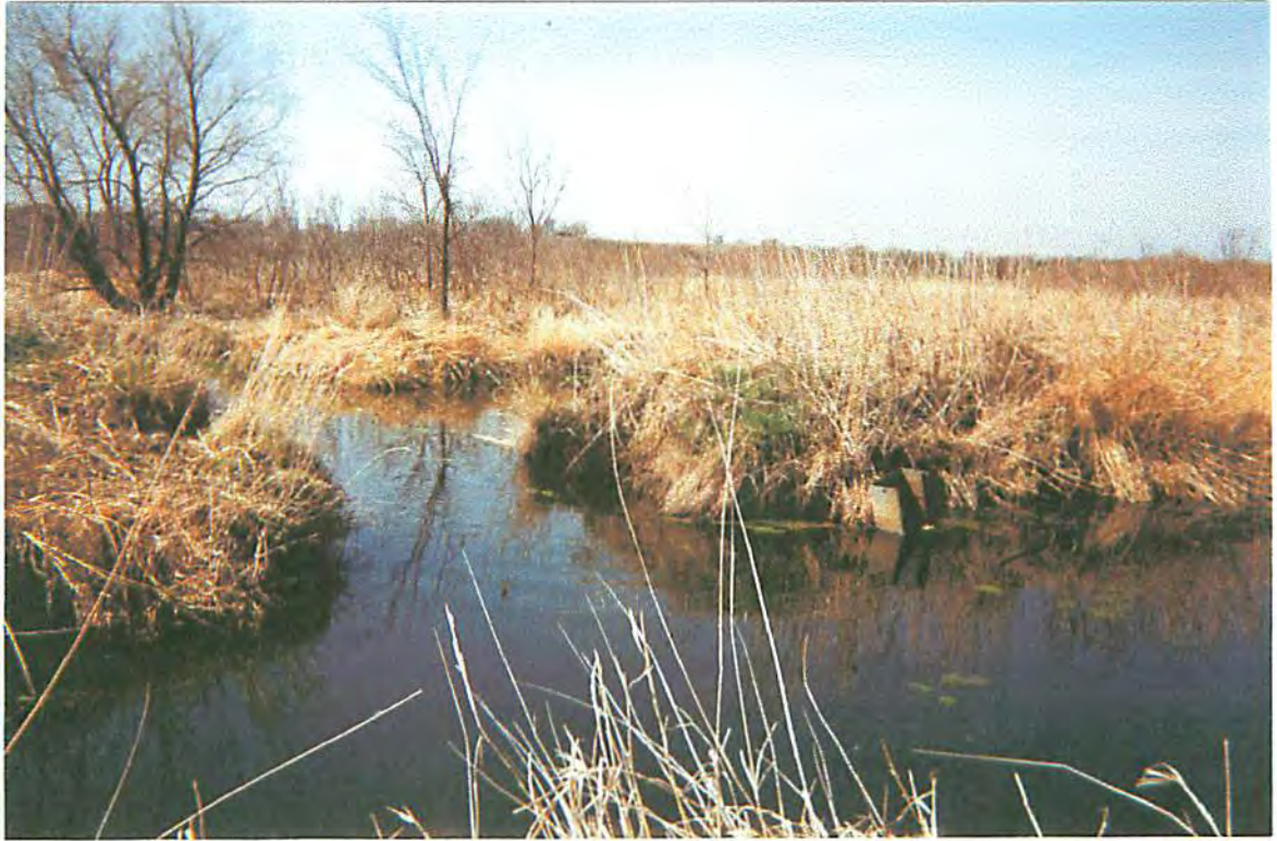
9. Kingston Wetland Treatment Project Berm Washout at West Overflow Structure.
