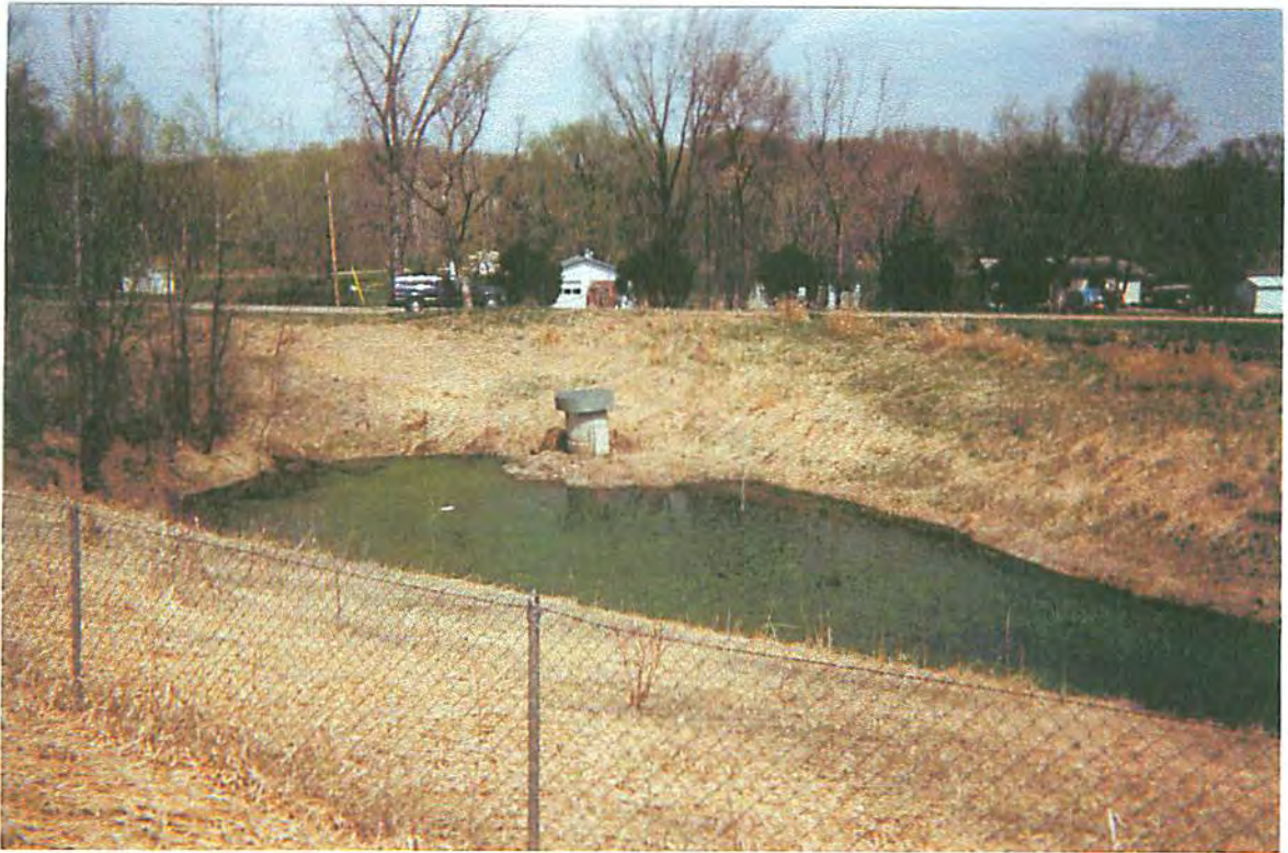
7. Lake Augusta Erosion Control Project. Sedimentation Basin and Overflow Structure.
