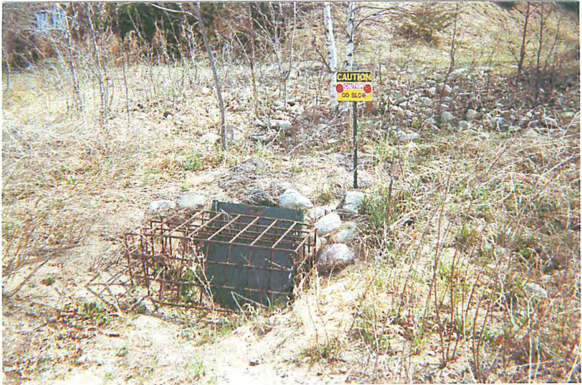
5. School Section Lake Outlet Project. New Outlet Structure.
