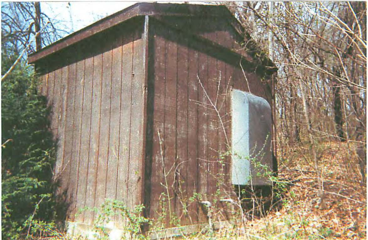
12. Aerator Building Lake Louisa.
