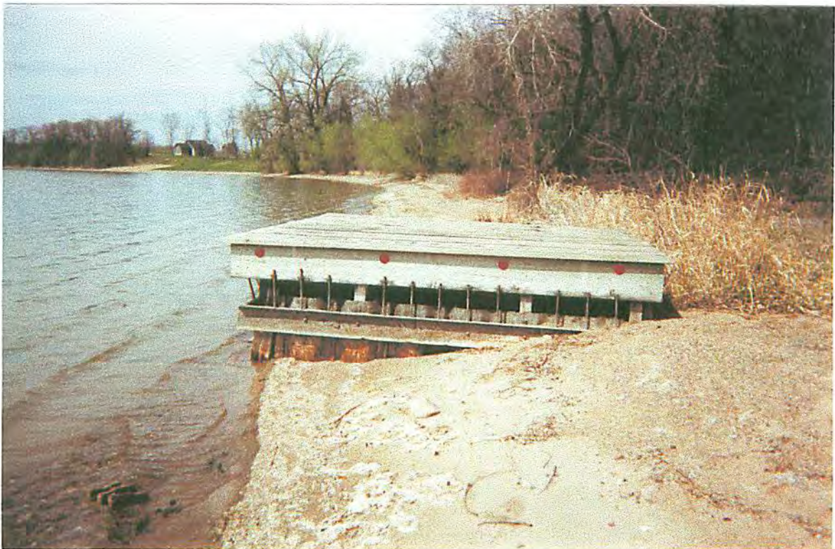
6. Pleasant Lake Outlet Project . Outlet Structure.
