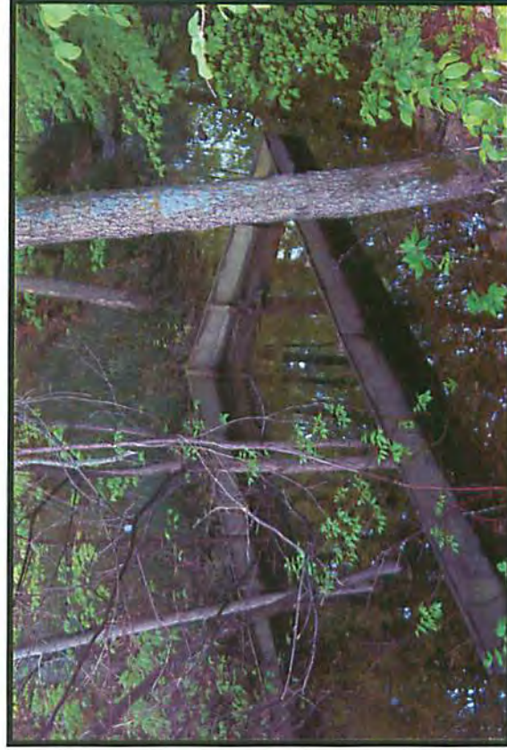
Photograph 12: Lake Augusta Erosion Control Project – west drop inlet structure.
