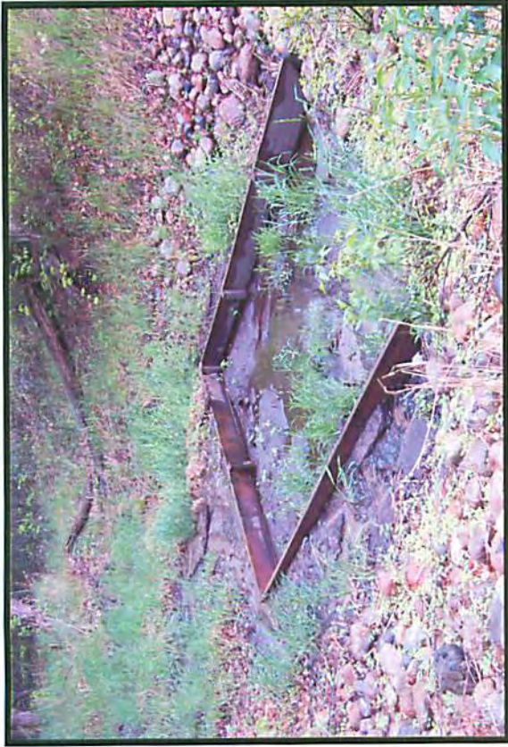
Photograph 13: Lake Augusta Erosion Control Project - south drop inlet structure.
