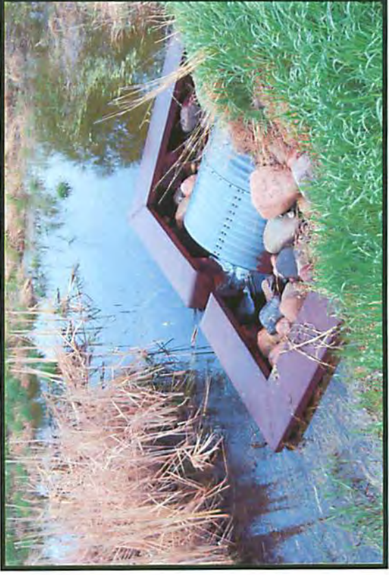
Photograph 14: Lake Augusta Erosion Control Project - sedimentation basin.
