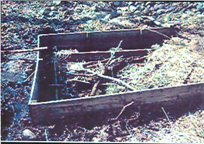
Photo 19 Lake Augusta Erosion Control Project - Inlet Baffles
