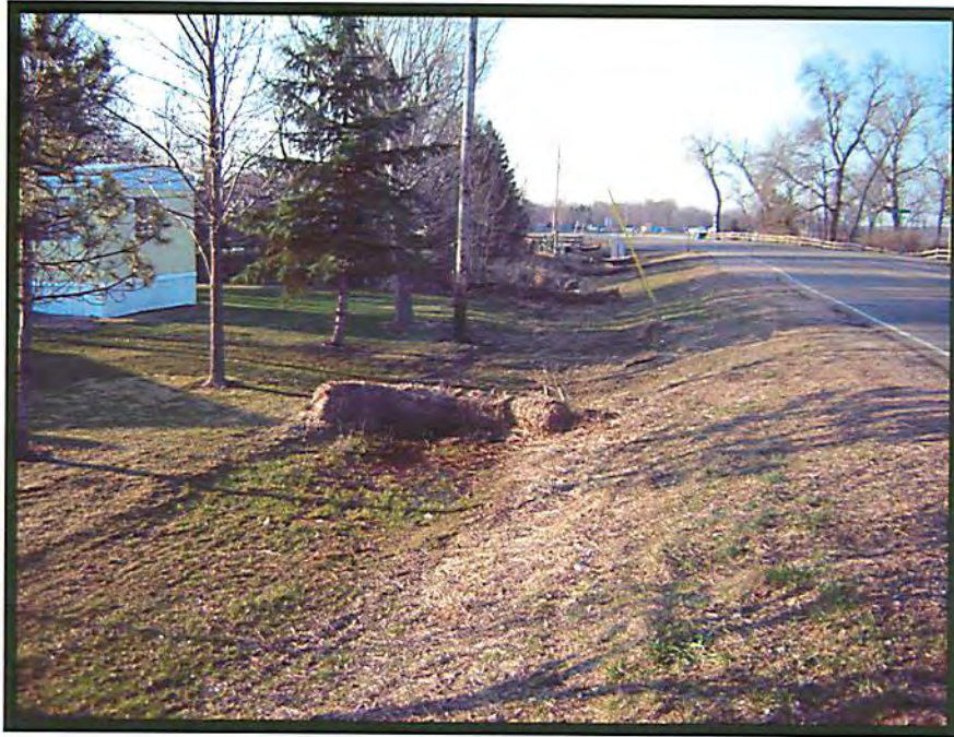
Photo 21 Clearwater Harbor Wastewater Collection and Treatment System (Remove check dam)
