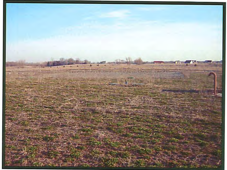
Photo 22 Clearwater Harbor Wastewater Collection and Treatment System (Drainfield)
