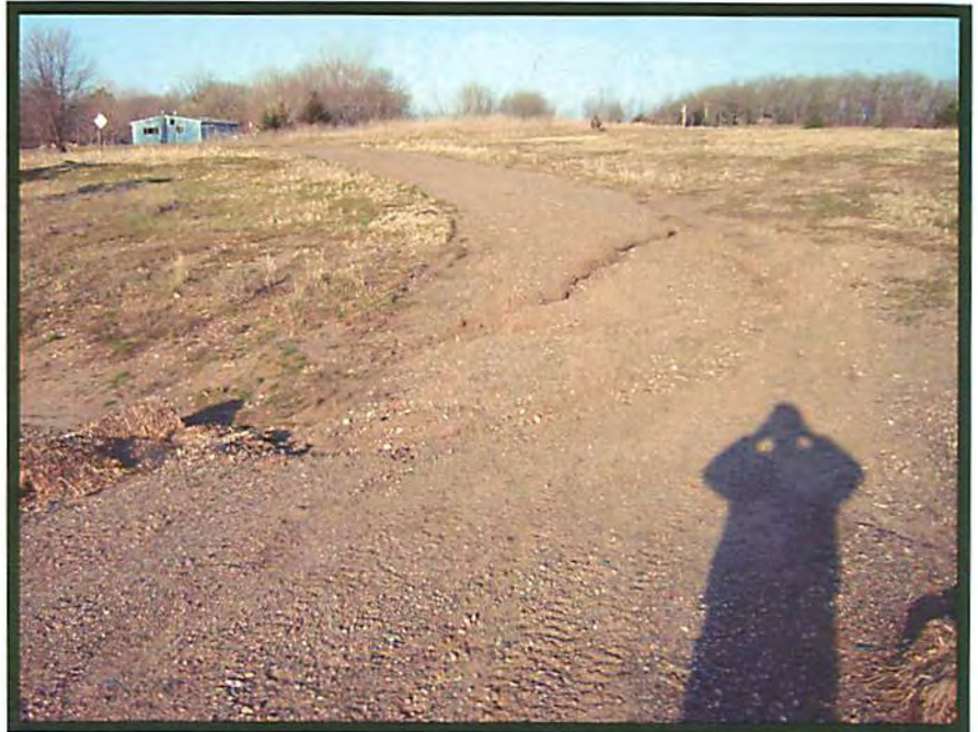
Photo 24 Clearwater Harbor Wastewater Collection and Treatment System (Erosion Repair)
