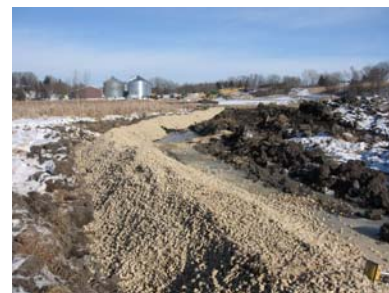
Segner Pond's limestone filter dike will remove additional phosphorus from water before it enters Cedar Lake.
