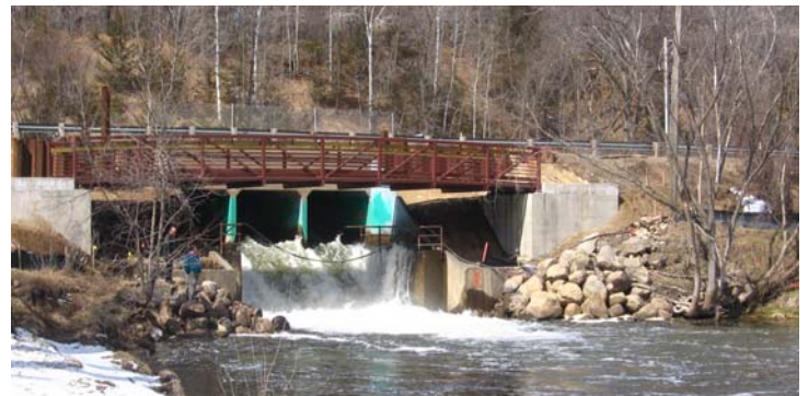
This dam on the Clearwater River just upstream from the Mississippi River marks the end of Clearwater River's reach. Two river stretches and 11 lakes in the CRWD have been listed as impaired by the MPCA.
