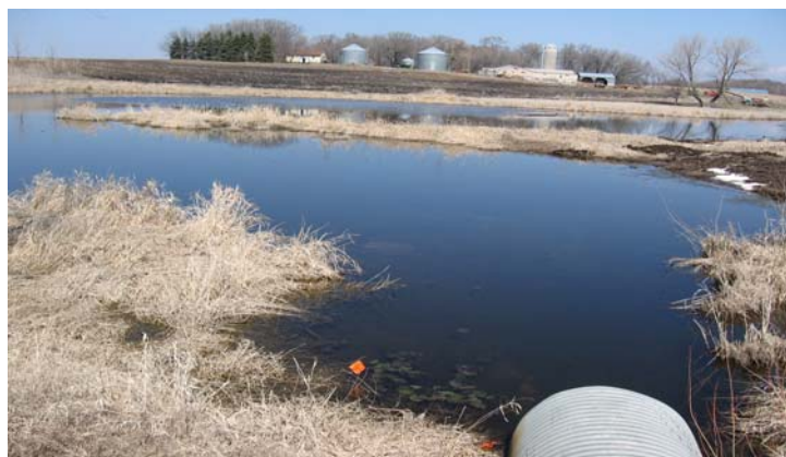
The Nistler/Geislinger sedimentation basin is one of many projects implemented on Clear Lake to improve water quality.
