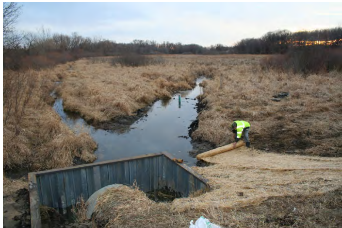
Constructed Notched Weir and Sand-Iron Filter
