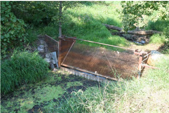
Fish Barrier at Illsley Ave.
