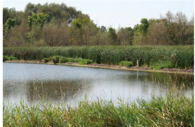
Segner Pond Limestone Berm Following Repairs
