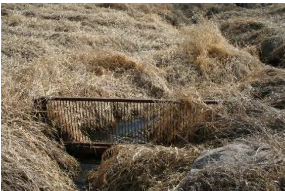
Fish Barrier at Henshaw Lake Outlet
