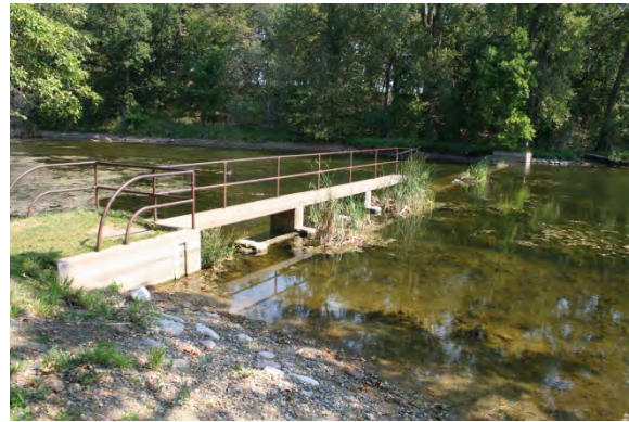
Grass Lake Dam August 31, 2012
