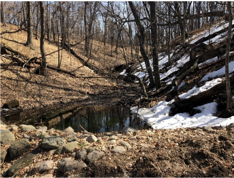
2019 Site Inspection. Erosion control channel + drop structure rip rap.
