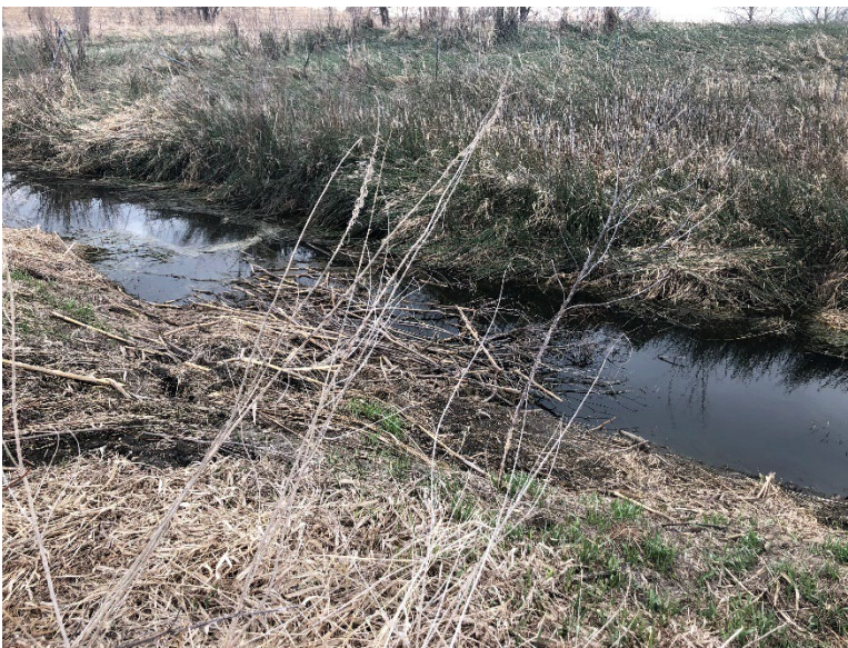
2019 site photo. Brush in diversion channel, with additional buildup would require cleanout
