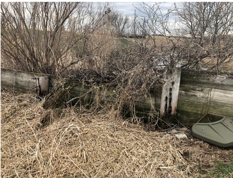
2019 Site Photos. Baffle berm, some burrowing by animals, brush needs to be removed
