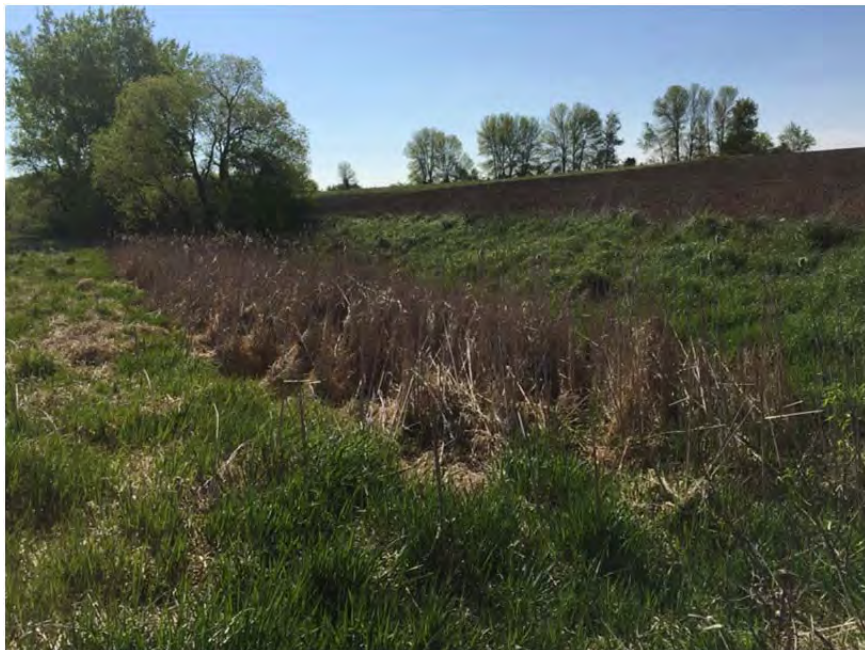
Cattails/Sediment blocking Channel B
