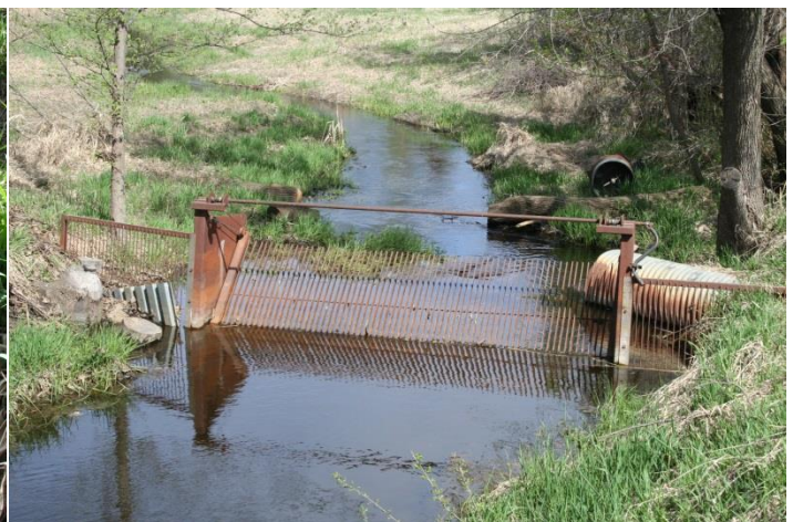
18-(Left) Temporary Repair at Illsley Ave Fish Barrier
