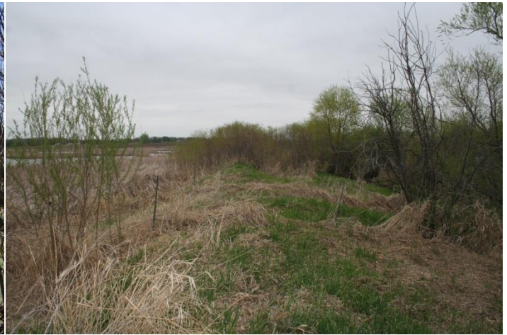
2-Brush/Trees on Berm at Watkins Isolation Project
