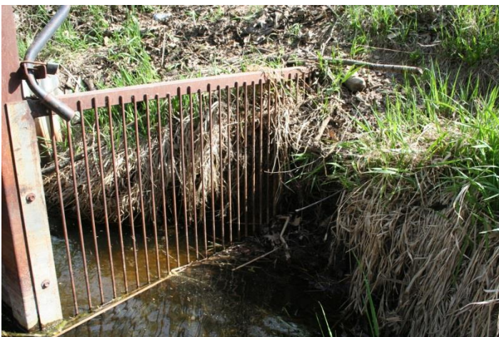
17-Eroding Bank at Illsley Ave Fish Barrier
