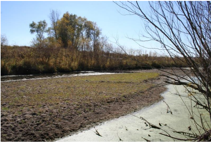
1-Sediment in Kingston Wetland Diversion Channel Basin
