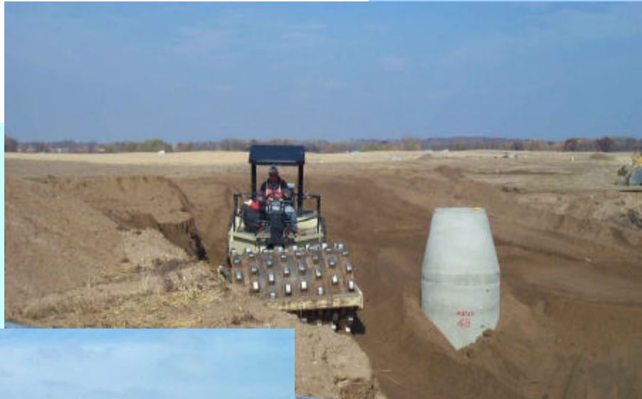
Installation of the sanitary sewer collection system
