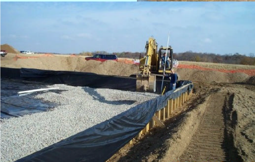
Installation of the wastewater re- circulating sand filter
